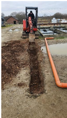
Deployment of pipes between raceway 1 & 2 for cables.
