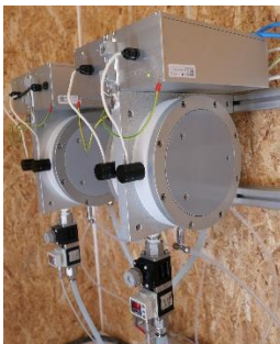
Gaia Ozone Generator WG120, Water ApS.
