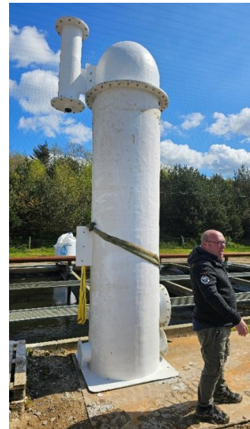
Vakuüm Air Lift (VAL 900, Coldep) on raceway 1.
