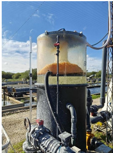
Skimmer (Ratz 950, CM-AQUA, TECHNOLOGIES ApS) on raceway 2.
