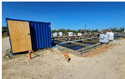
Buried conduits used to protect power and data cables from damage associated with routine operations at the trout farm.
